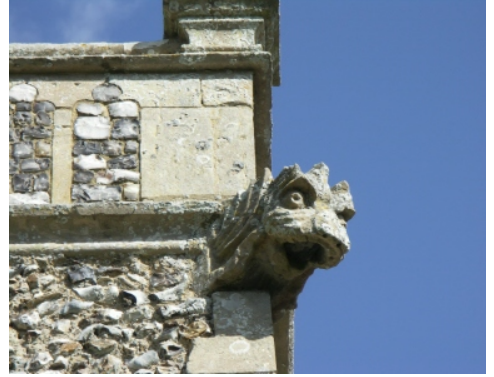
Gargoyles are fascinating details along the parapets of a church but their primary role was just to throw water off the roof so it did not damage the wall and foundation below.
